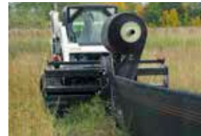
Silt Fence Installer on page 90
